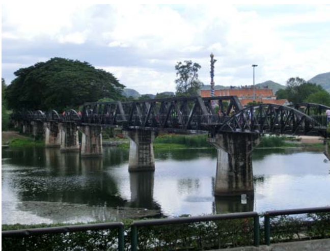
The center two trapazoidal spans of the Kwai river bridge are the bombed out replacements constructed after the end of the war, the rest of the spans are original construction.
