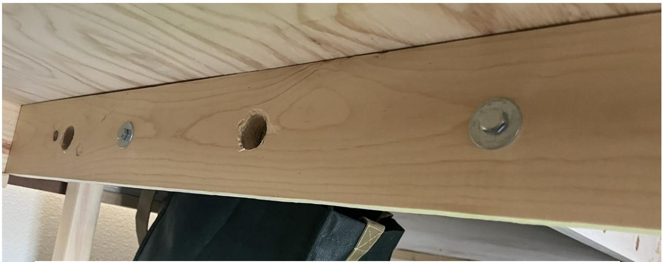
***Figure 9 Underside of benchwork with screws and holes for wires.***
